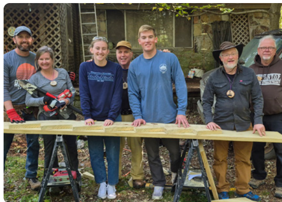
Mountain T.O.P. volunteers repairing the front steps for a F@H member, making it safer. Thanks, Mountain T.O.P.!
